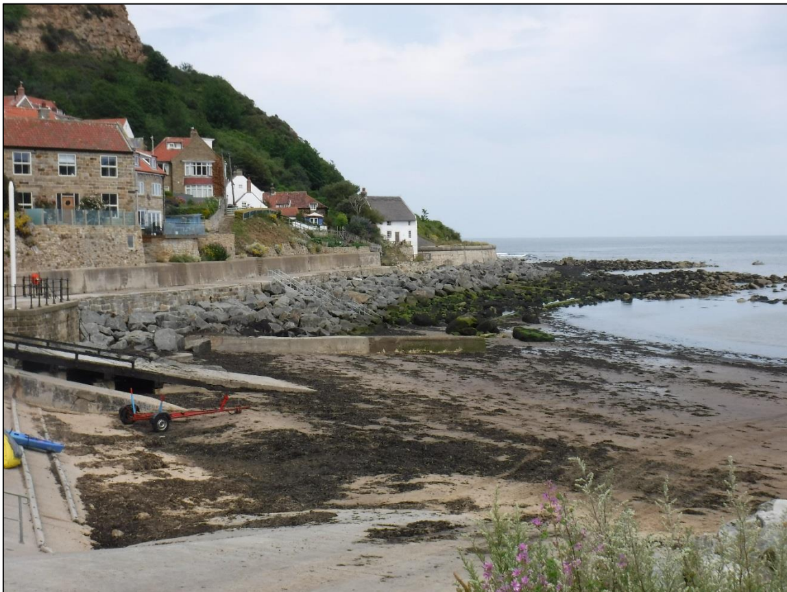
Figure 2.1. Location of new granite rock armour at the foot of the seawall, note the green (colonised) natural boulders which have been placed in front of the granite rock (July 2019).
